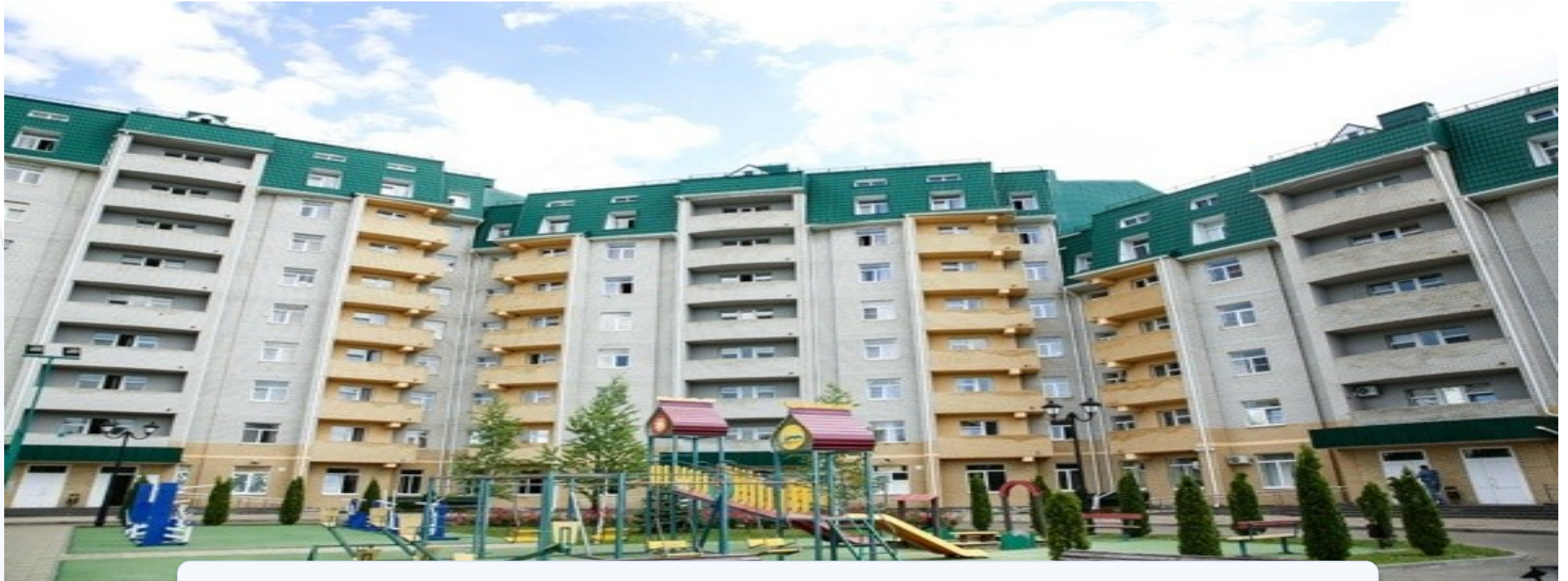
Dormitory No. 5, No. 6 and No. 7 — Address: 2 Kulakova Avenue, Stavropol
